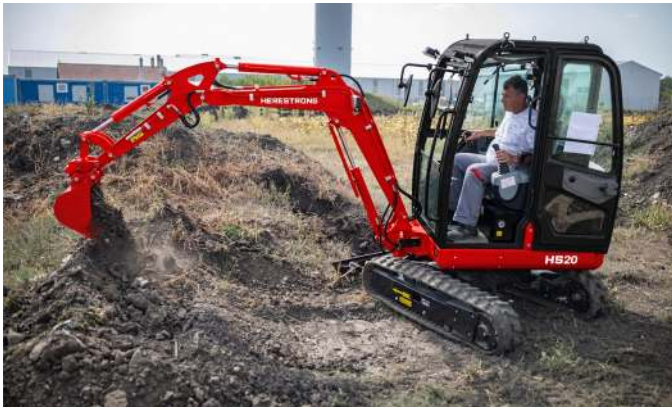
HS20 in Germany — site cleanup
